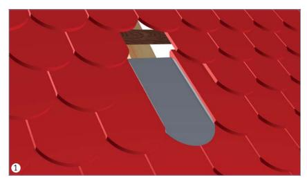
Remove the plain tile, where the roof hook will be placed, and also surrounding tiles.
